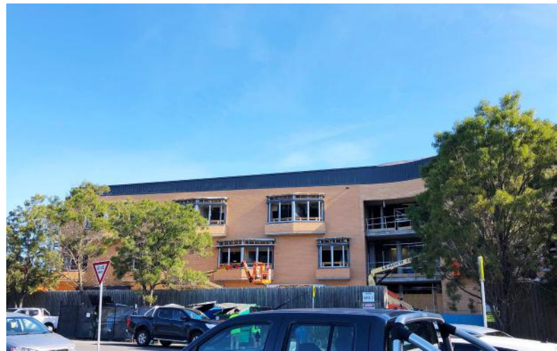
Progress (pictured, above) of the Avondrust Lodge re-development project.
